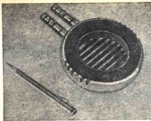
Above—Lower bars of Schlieren-optic with water cooling. Upper right—Rotating glass plate which carries the light-control fluid. Lower right—Upper bars of the light-control.
